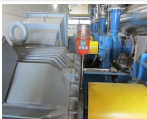
14 units of Pulsarlube M 125cc installed in Compression process
